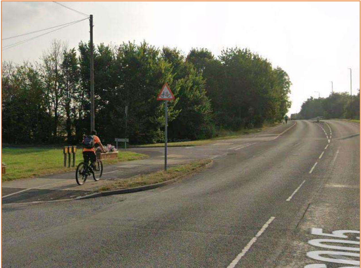
Figure 11: Cycle track alongside the A6005 looking east towards the M1 bridge.
