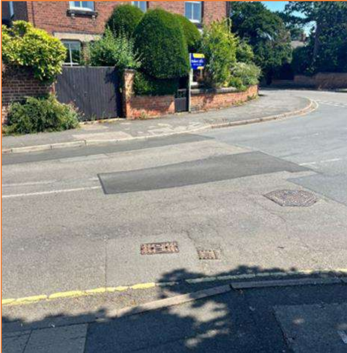
Figure 7: Crossing on Stevens Lane
