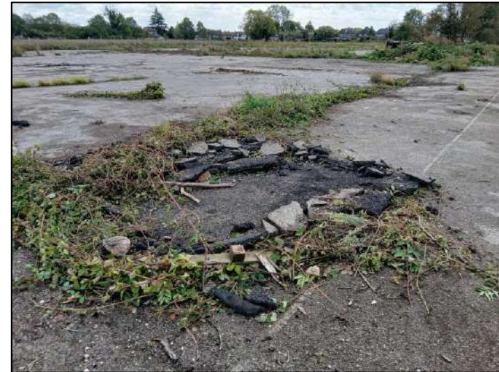
Photo 12 - Exposed Tarmac in North-Eastern Area
