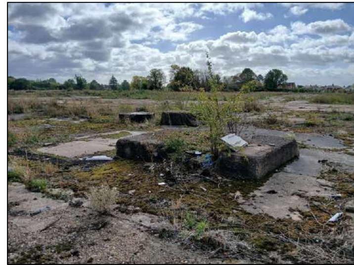
Photo 6 - Remnant Concrete Pads / Blocks
